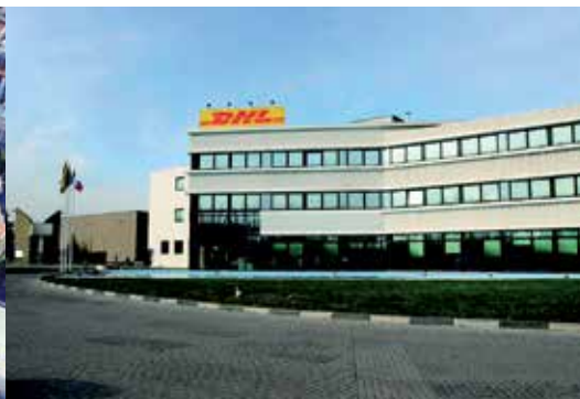
DHL - Data Center - Italy
